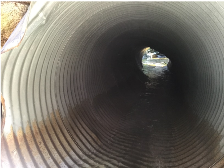
Looking through downchain culvert
