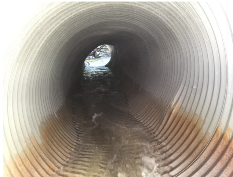
Looking through upchain culvert
